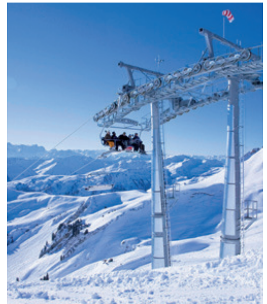
Tower group with sheave assemblies and carrier of a circulating passenger ropeway type 6-CLD
